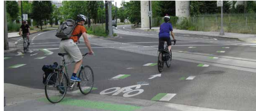
Example of a bicycle/pedestrian only phase with a diagonal bicycle/pedestrian crossing. NE 201st Avenue currently does not have on-street bike lanes north of NE Halsey Street; therefore, this improvement should be tied to improvements along NE 201st Avenue and/or installation of an off-street trail system.
