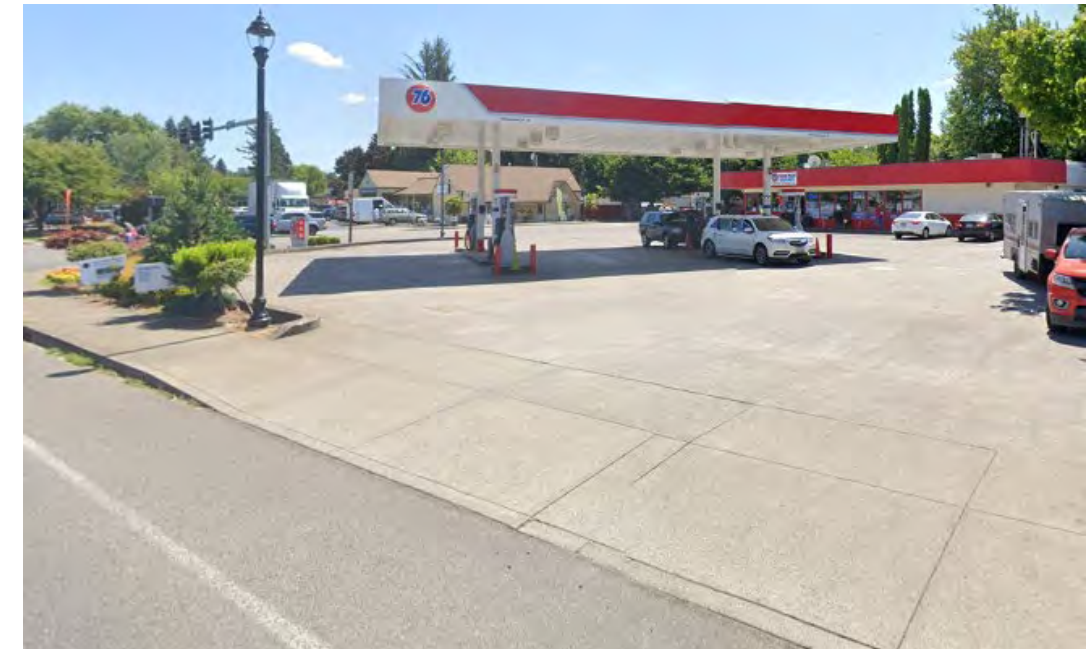
Gas station at 238th/Halsey
