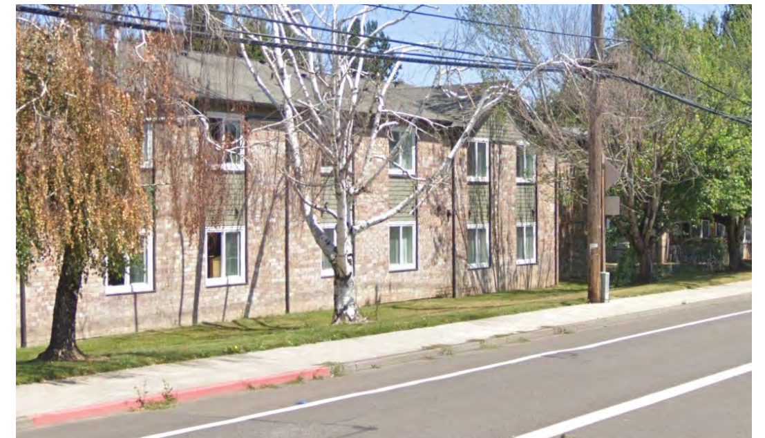
Housing on the ground floor with no entrances facing the street
